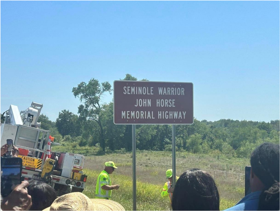
Oklahoma DOT erecting Seminole Warrior John Horse - Memorial Highway Sign
